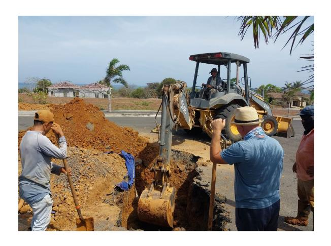
The drain between lots 6 and 7 was completely blocked and the drain across from lot 5 was completely clogged. A water trench diversion was dug behind lots 23-27. Drainage covers were replaced in the street.
