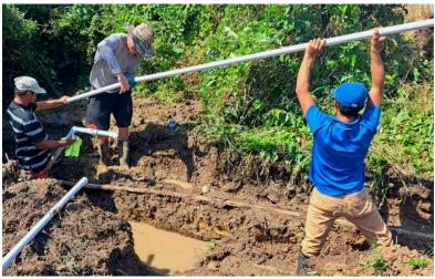
The pipe leaking by casa 60 has been repaired. The hole has been backfilled and the road will be repaired when backfill has settled.
